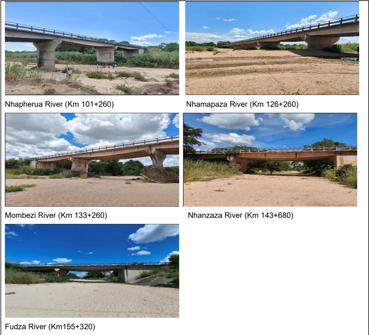
Figure 4 Pictures of existing bridges Km 84-168 captured by design consultant, LASA, March 2024 Source: Inception report, LASA, March 2024
