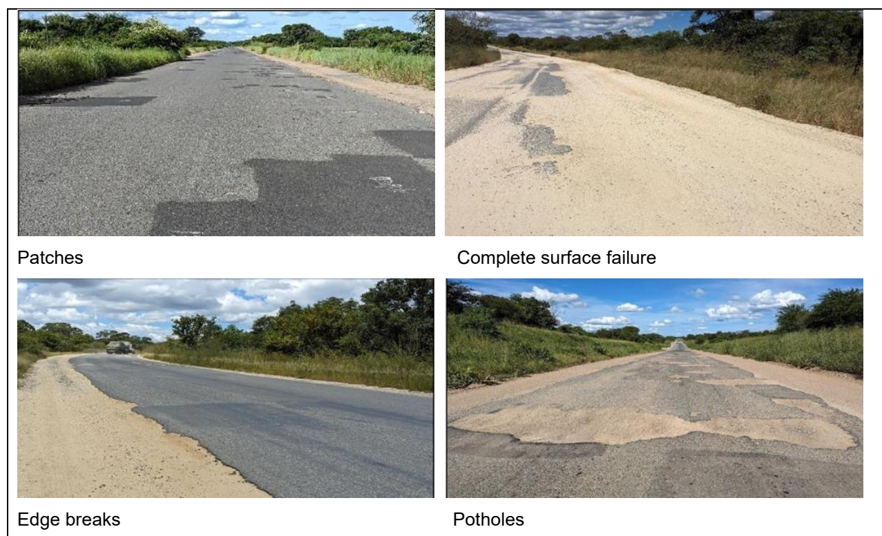
Figure 6 Existing pavement conditions noted by design consultant LASA, March 2024
