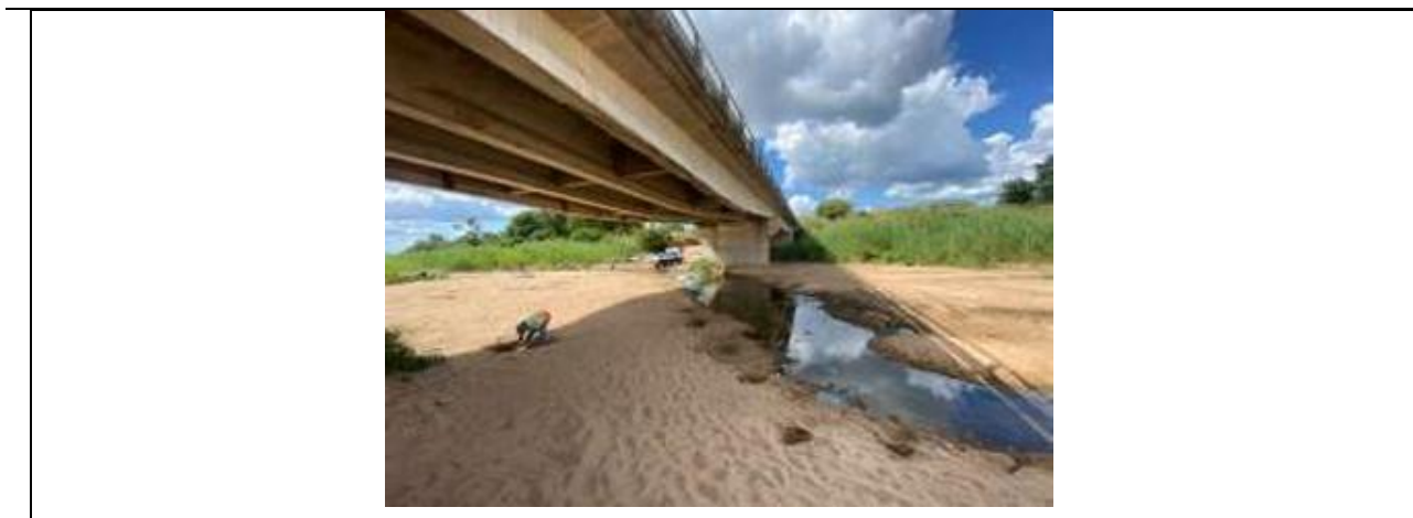
Figure 11 Images of water source identified by design consultant LASA, April 2024
